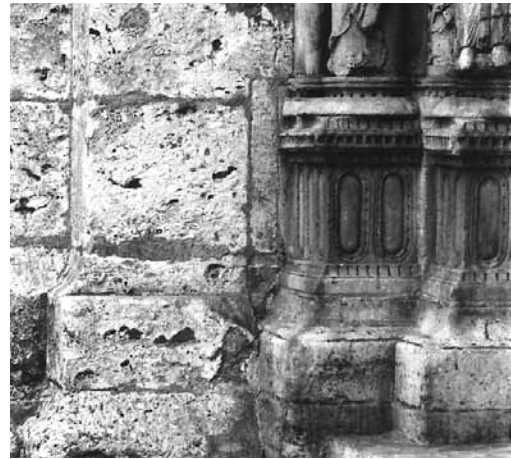
North plinth against the tower
