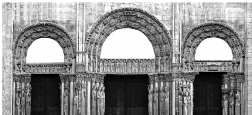
Proposal for the portal in campaign F in 1139. Round arches over single lintels
