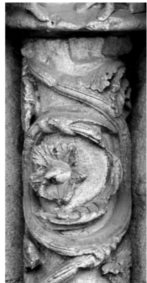
9 - cr2t by Héron was carved in group 2. It was cut short at both ends in campaign I that left it 127cm long. It looks like the cutting was crudely executed. This is one of the longest of the shortened shafts.
