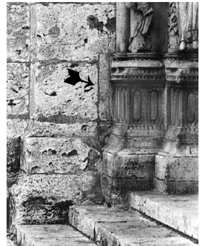
Cut into the north tower to insert the plinths in E
