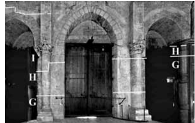
Interior of portal with campaigns marked
