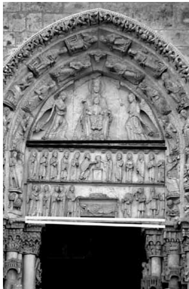
Gaps between lintels and tympanum adjusted
