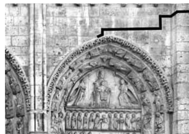
Bonded coursing from tower to apex of south portal
