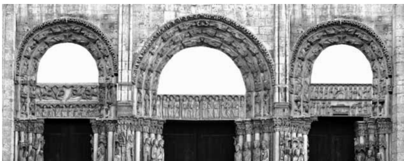
Proposal for the portal in campaign G in 1140, and continued in H. Round arches over doubled lintels
