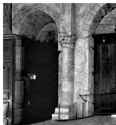
Interior wall of portal with attached shaft
