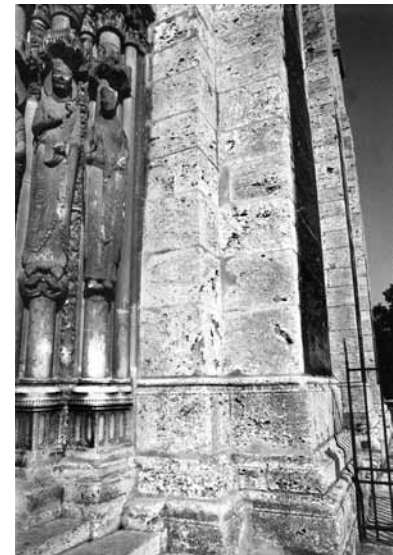
Bonded junction between south portal and tower
