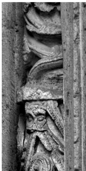
10 - bottom of '9' cr2t by Héron over Longleaf, carved in group 2 and cut back at both ends in campaign I. Though hard to see in a narrow space between the figures, the different stones and the incomplete forms in the upper shaft highlight the junction.
