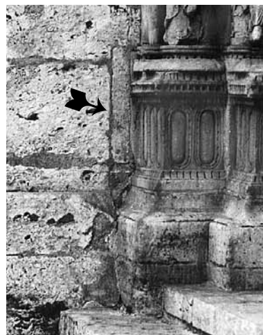
Breaking into north tower for the portal plinths
