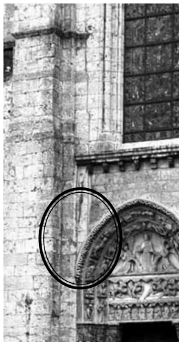
Junction north portal and tower
