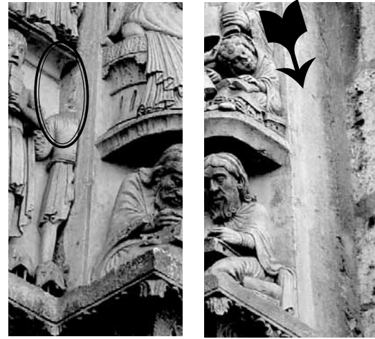
South portal, the differing infills next to the lintels
