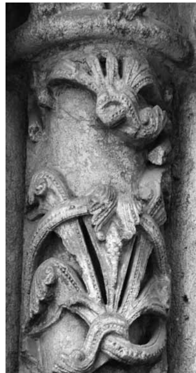
1 - nL2t by Héron carved in group 2. It is 0,78cm high. Truncated by slicing through one of the bouquets at the top and placed by G when he finalised the door height and placed the capitals over the left jamb.
